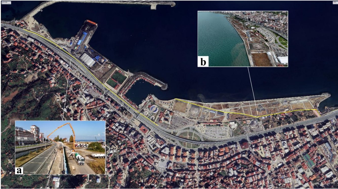
Figure 2. Bicycle Paths Under Construction. a) Bicycle path under development between the Police Social Facility and the Tea Market (Çay Çarşısı). b) Bicycle path under construction within the Nation's Garden (Millet Bahçesi).
